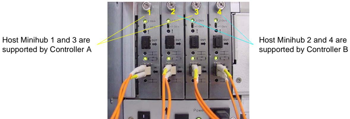
**Note:** Storage systems that use the model 28xx controllers will have host and drive interface ports on the controller FRUs, as shown below. The left FRU is Controller A and the right FRU is Controller B. Refer to the Array Module manual for more information.
