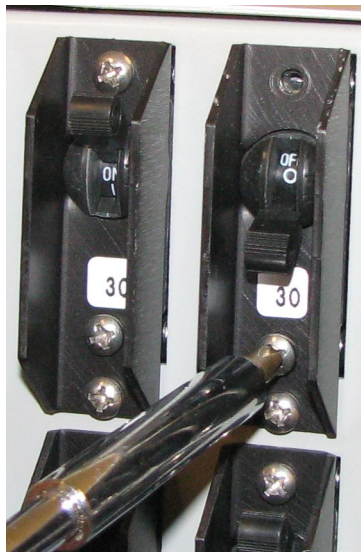
Figure 9: Unscrew the Breaker
