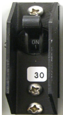
Figure 15: Push Breaker to ON Position
