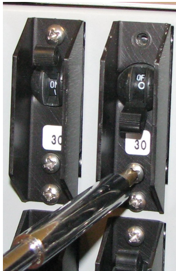
Figure 15: Push Breaker to ON Position
