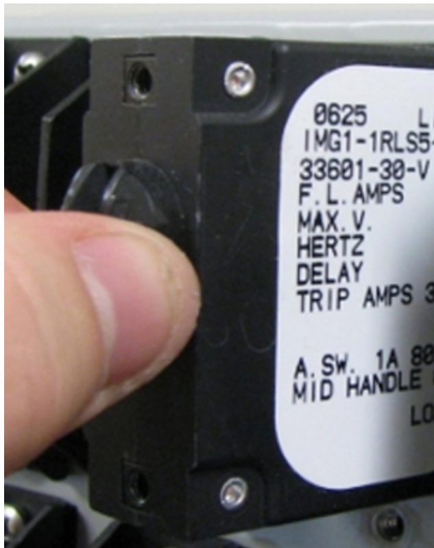
Figure 11: Remove Breaker
