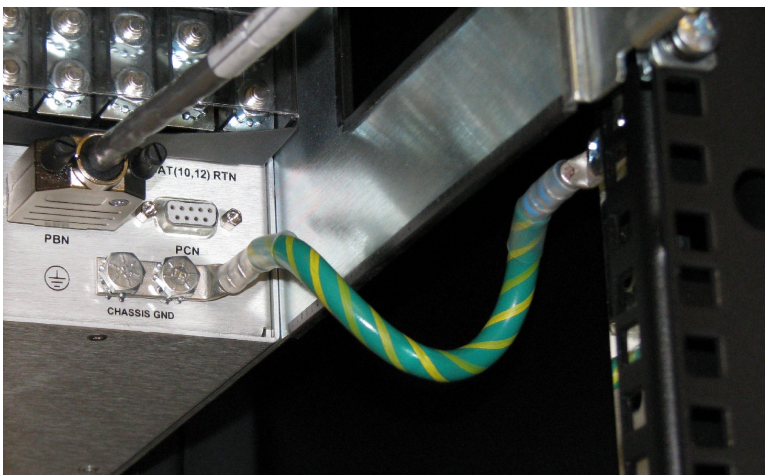
Figure 33: Grounded PDP
