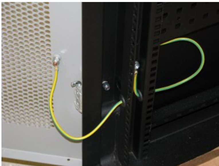
Figure 32: Door Ground - Top
