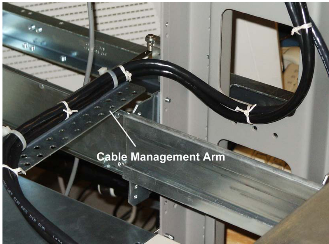
Figure 53: Side Cable Management Arm Installation
