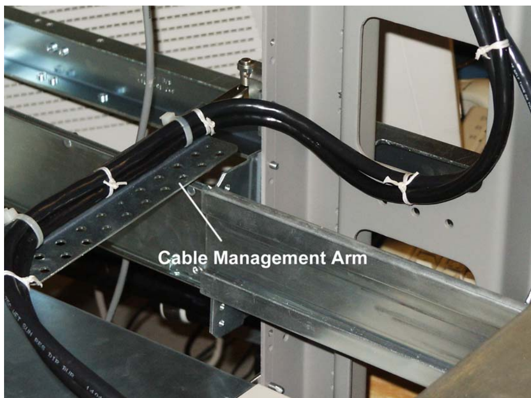
Figure 5-9. Detail of a Side Cable Management Arm
