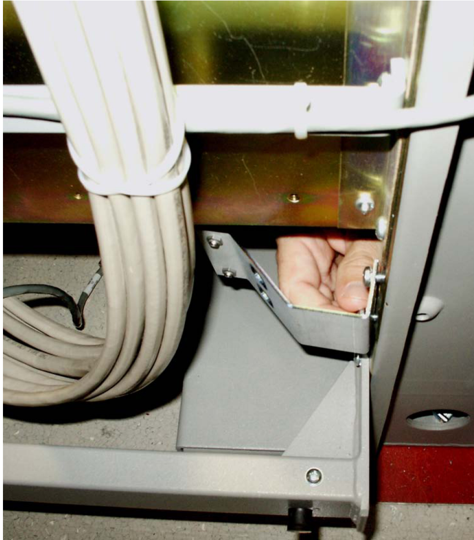
Figure 82: Attach side fan bracket to front frame rail
