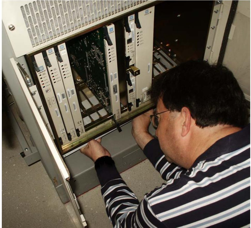
Figure 6-17 Insert fan tray bracket
