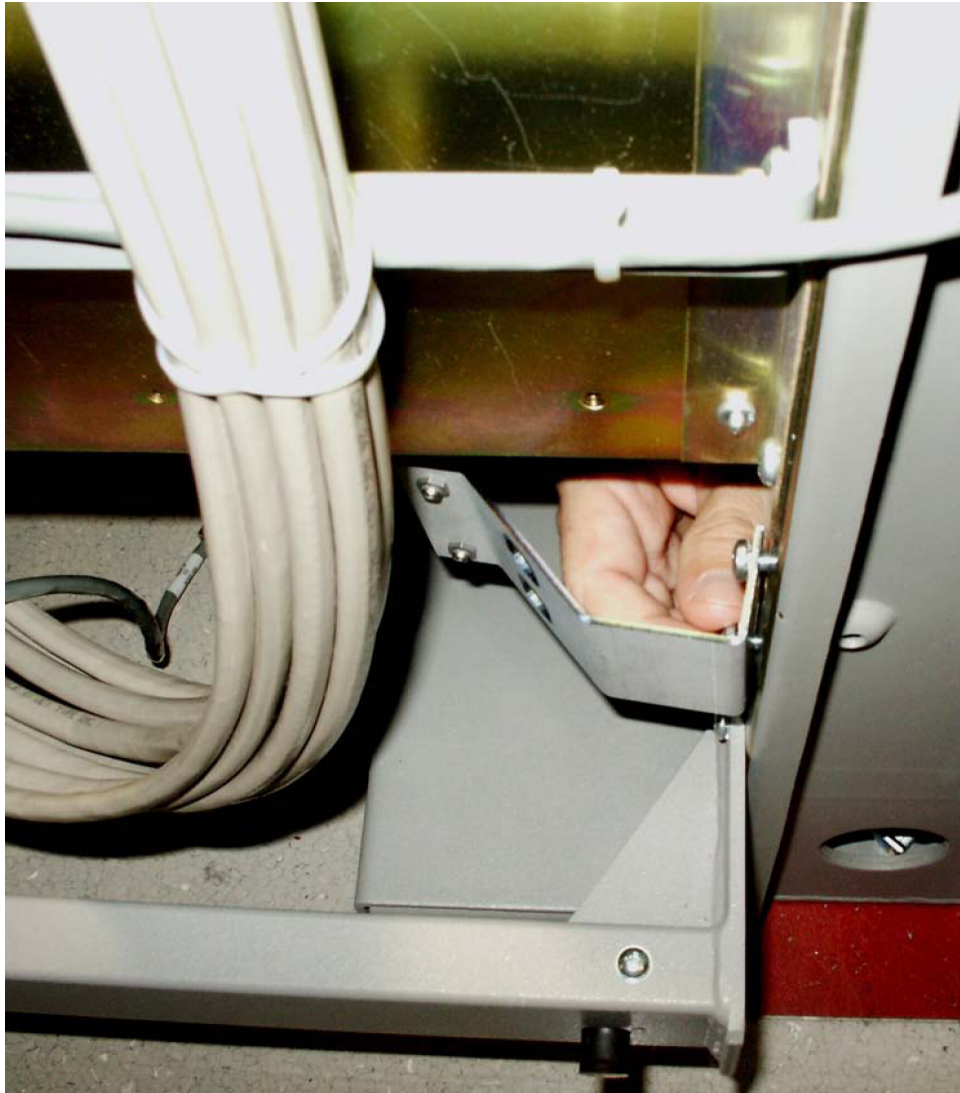
Figure 6-14 Attach side fan bracket to front frame rail
