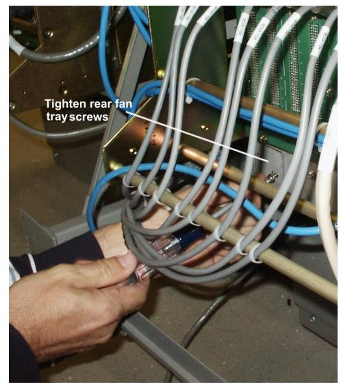
Figure 6-21 Tighten rear fan tray screws
