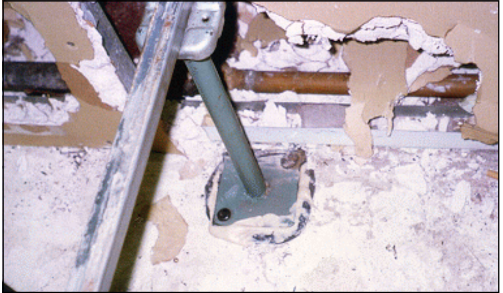
FIGURE 3-6 Subfloor Penetration
