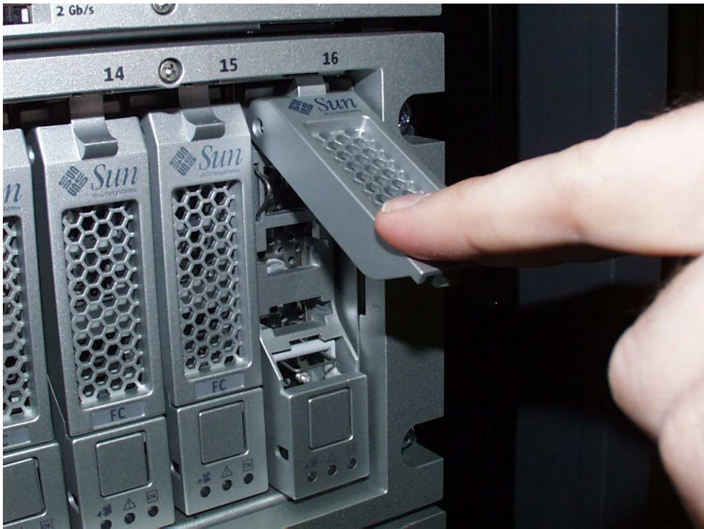
FIGURE A-2 Successfully Inserted Disk Drive
