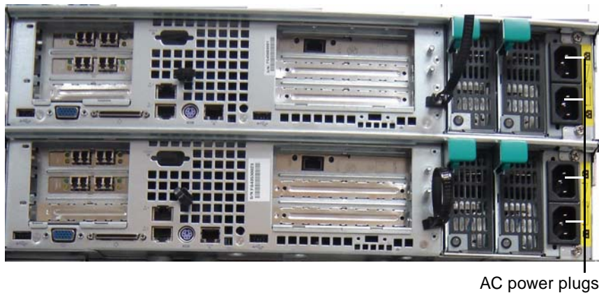
FIGURE 3-23 Connecting the Sun StorEdge 5310 Cluster AC Power Cables
