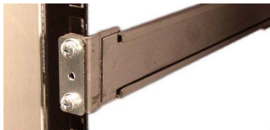
Figure 2 - 47. Stationary Slide Securely Attached to the Equipment Rack
