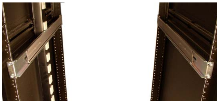
Figure 2 - 45. Stationary Slides and Extenders Installed in Equipment Rack
