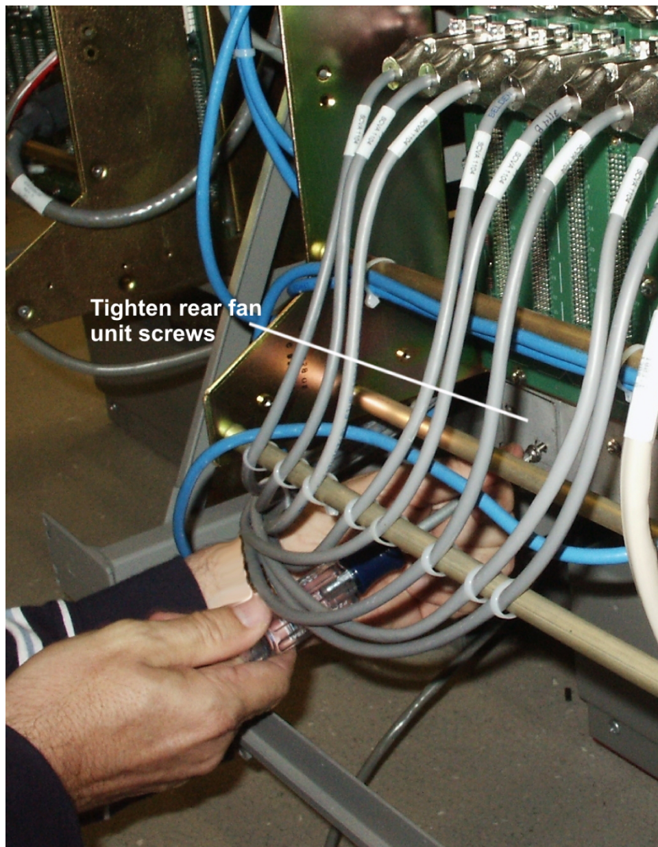
Figure 65: Tighten rear fan tray screws
