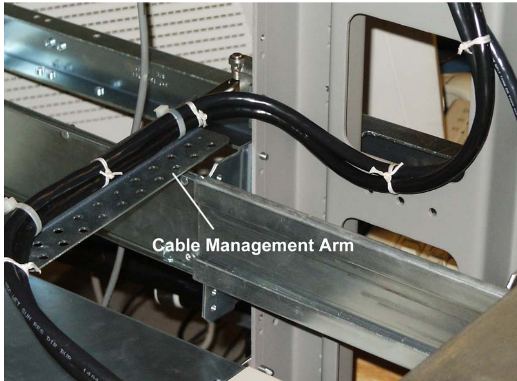
Figure 5-9. Detail of a Side Cable Management Arm
