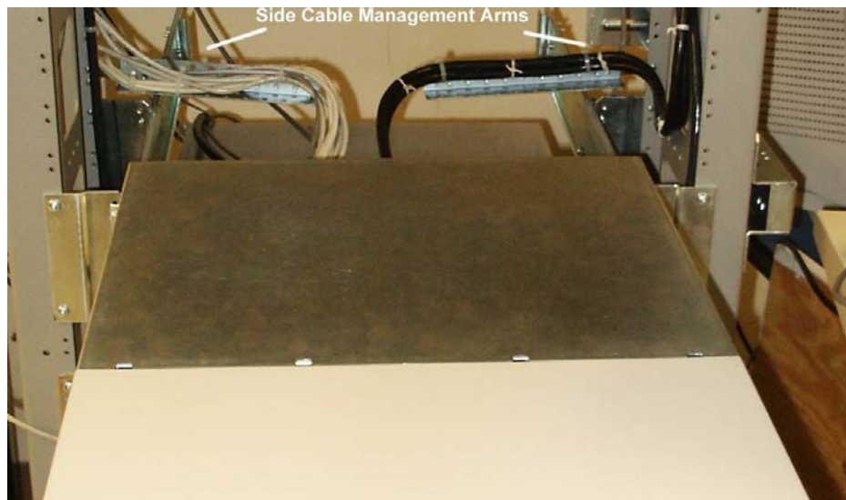
Figure 3-6. T1100 AS with Side Cable Management Arms
