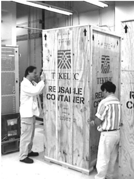
6.) CAUTION: To avoid injury or damage to equipment, this step requires two people. Lift front panel out and away from crate.
