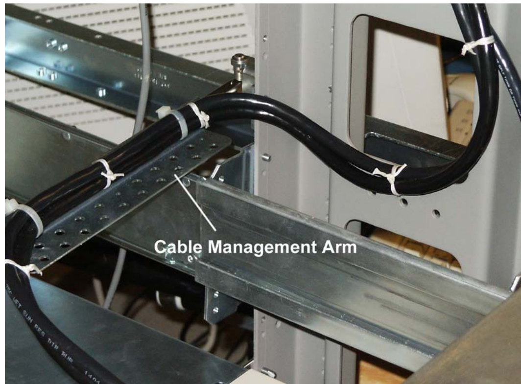
Figure 5-9. Detail of a Side Cable Management Arm
