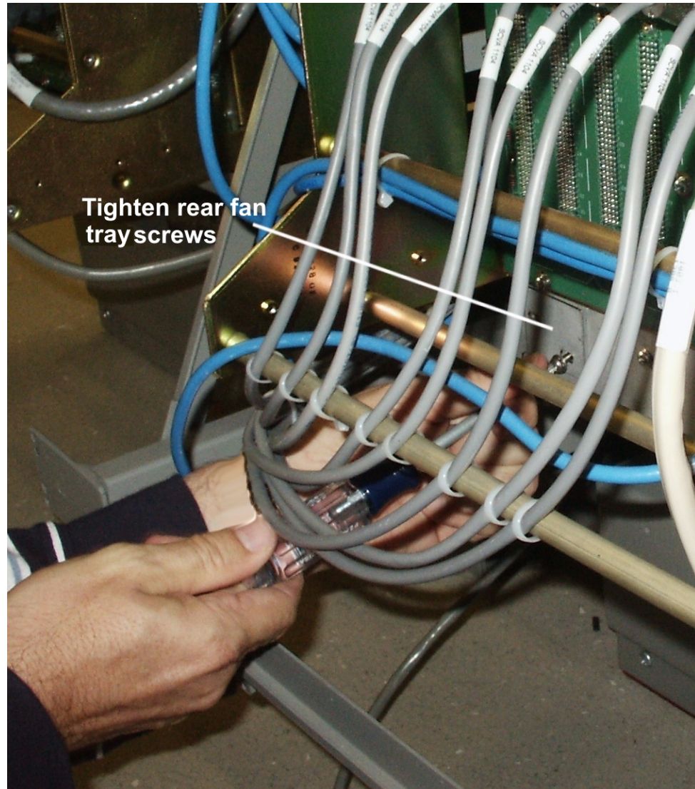
Figure 6-21. Tighten rear fan tray screws
