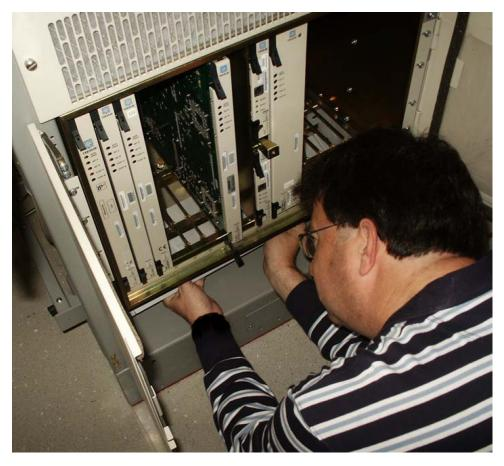
**Note:** When inserting the fan tray bracket, be sure not to pinch cables between the bottom of the shelf and the fan tray bracket.
