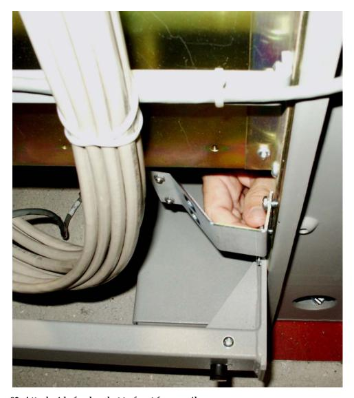
Figure 82: Attach side fan bracket to front frame rail
