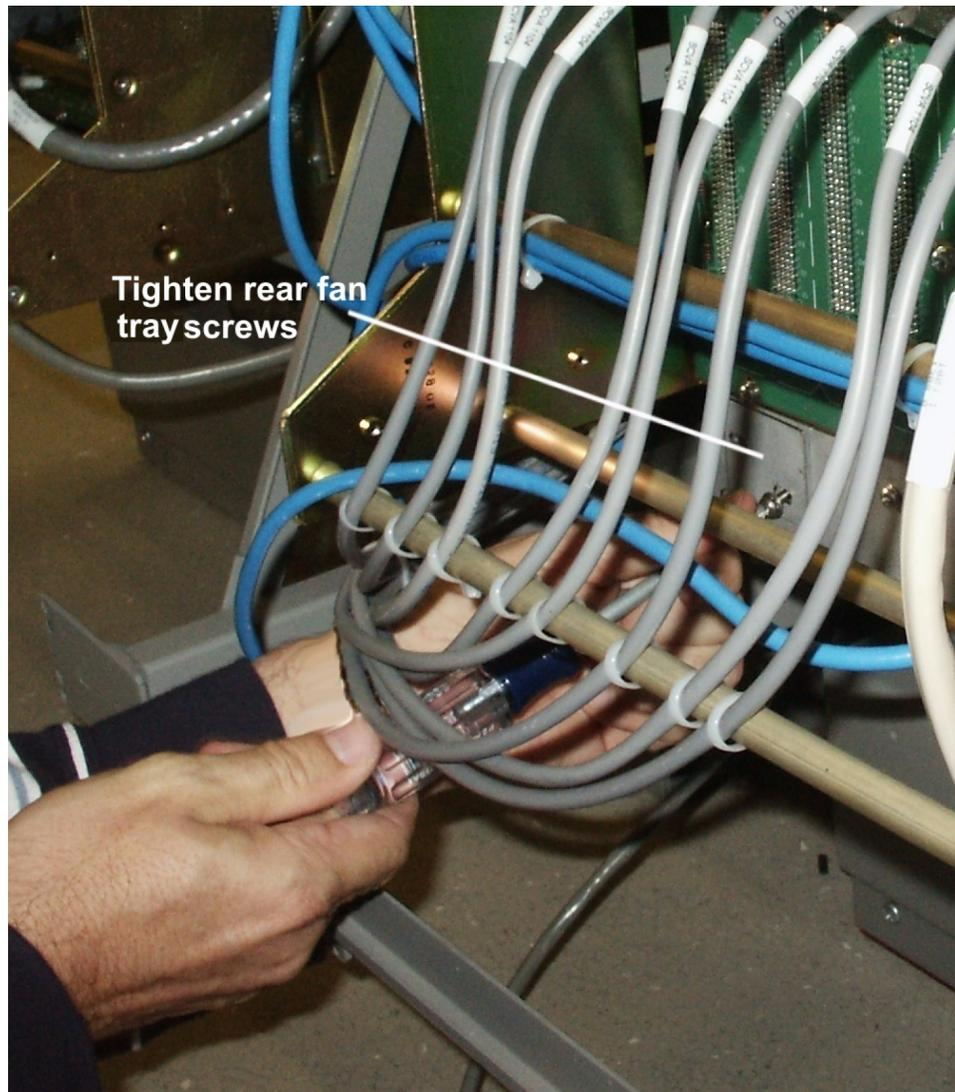
**Figure 89: Tighten rear fan tray screws**
