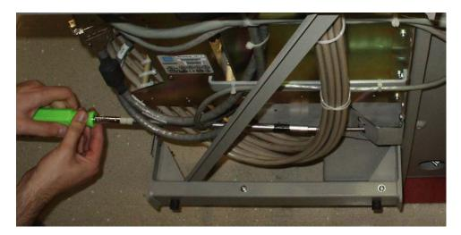
Figure 90: Tighten fan side bracket screws
