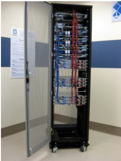
Figure 44: Example of T1200 cabinet with Pre-cabled Components
