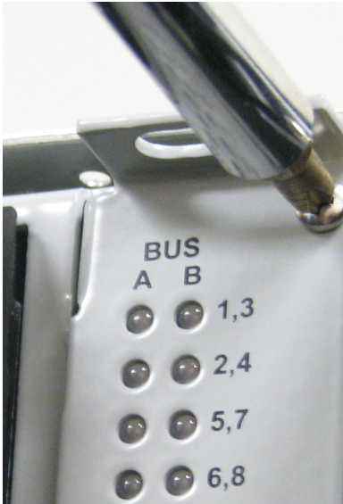
Figure 37: Unscrewing Alarm Card
