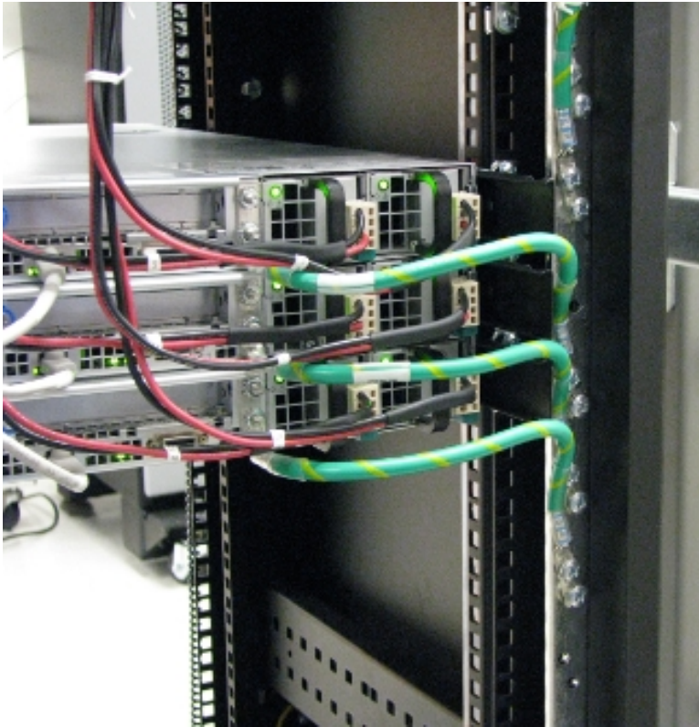
Figure 34: Grounded T1200 Application Server
