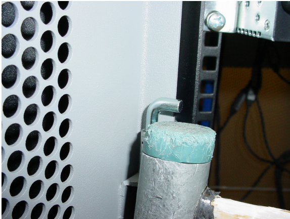
Figure 29: Removing pin with rubber hammer
