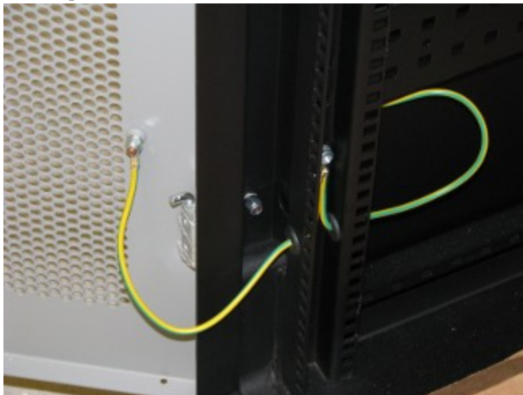
Figure 31: Door Ground - Bottom
