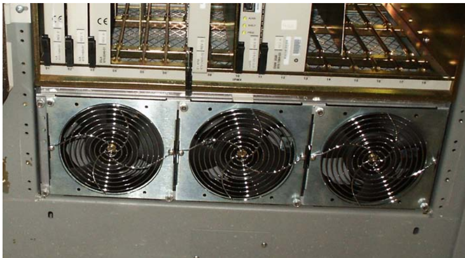
Figure A-28.Fan tray inserted into fan tray bracket in the frame - front view
