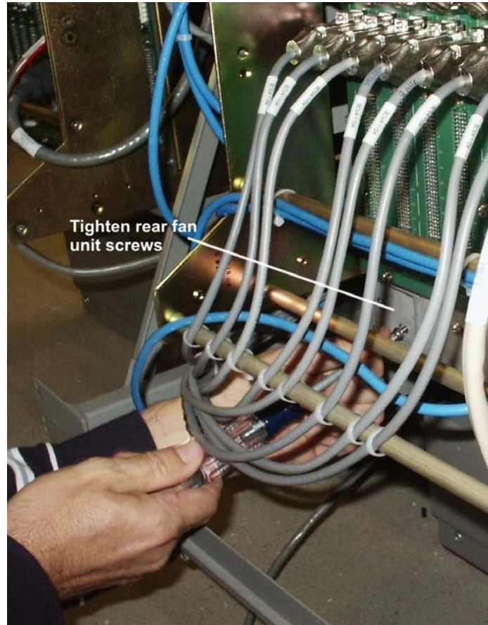
Figure A-29. Tighten rear fan tray screws
