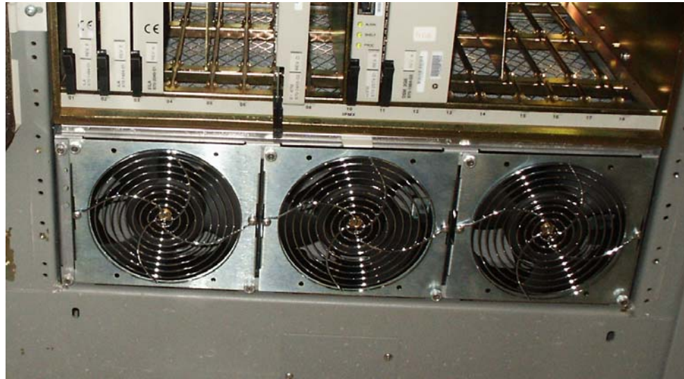
Figure 5-20. Fan tray inserted into fan tray bracket in the frame- front view
