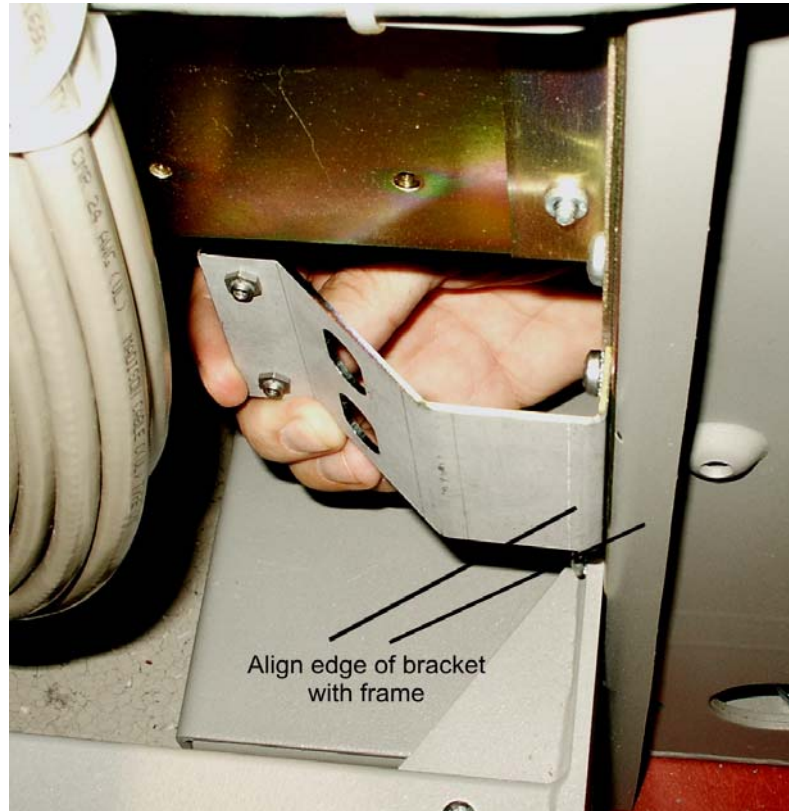
Figure 5-15. Slide the side fan brackets flush with the Frame
