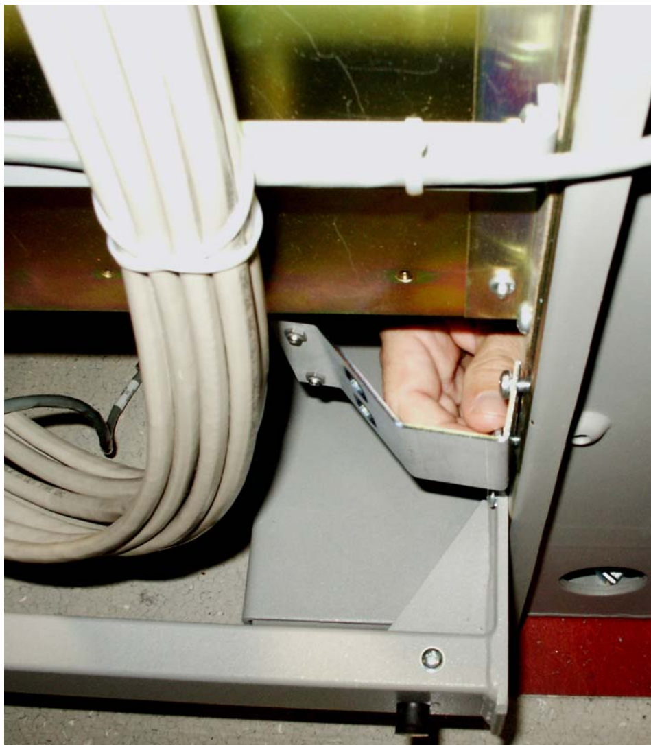
Figure 5-14. Attach side fan bracket to front frame rail
