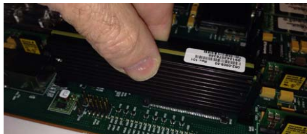
Figure 6 - 119. Removing the Transcoder DSP Module
