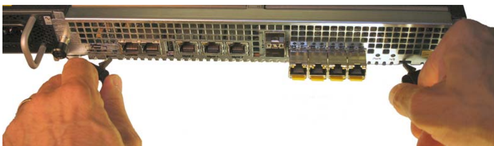
Figure 6 - 107. Installing the NIU
