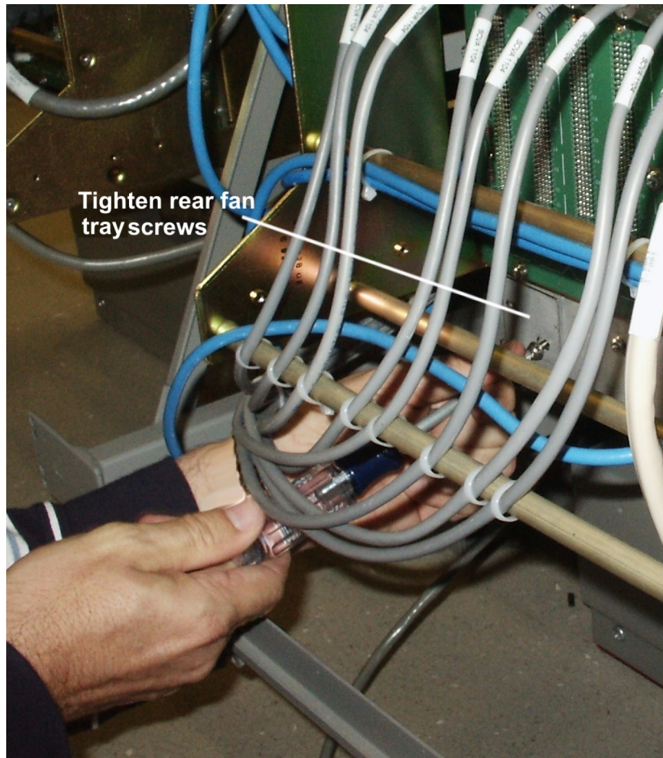
Figure 89: Tighten rear fan tray screws
