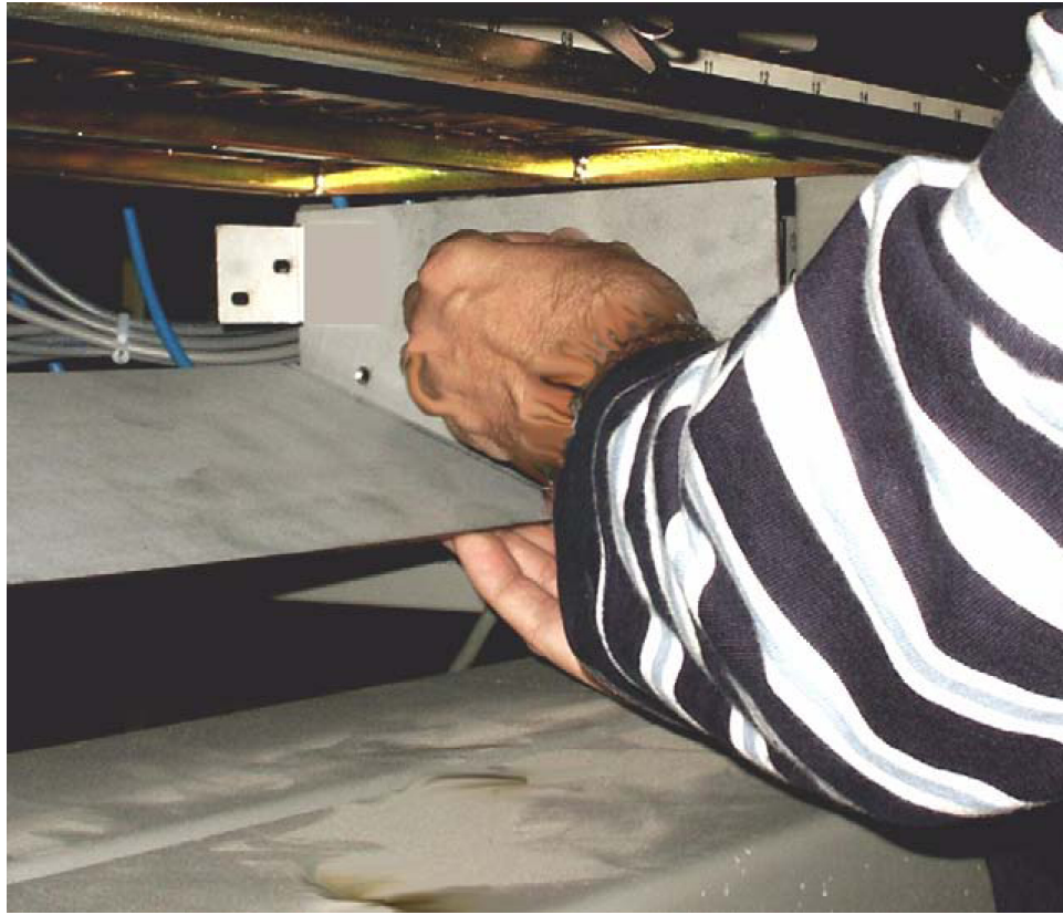
Figure 86: Attaching the fan tray bracket to the side brackets - inside front
