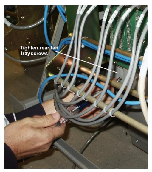
Figure 89: Tighten rear fan tray screws
