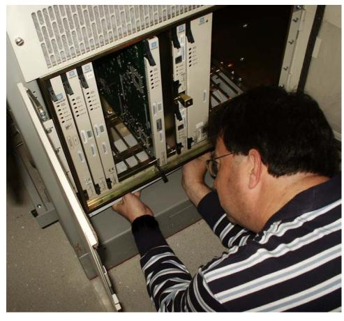
**Note:** When inserting the fan tray bracket, be sure not to pinch cables between the bottom of the shelf and the fan tray bracket.
