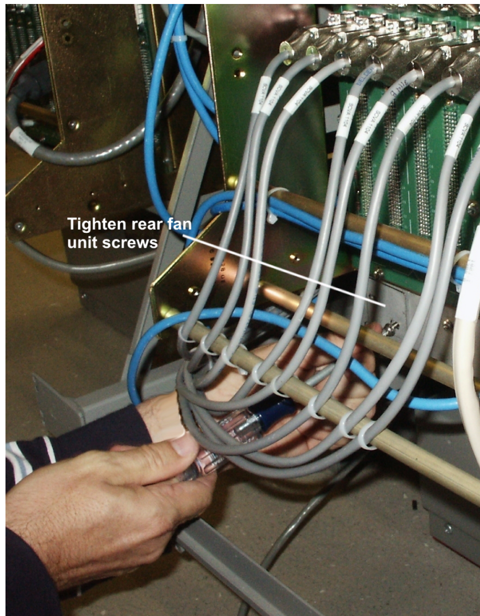
Figure 47: Tighten rear fan tray screws
