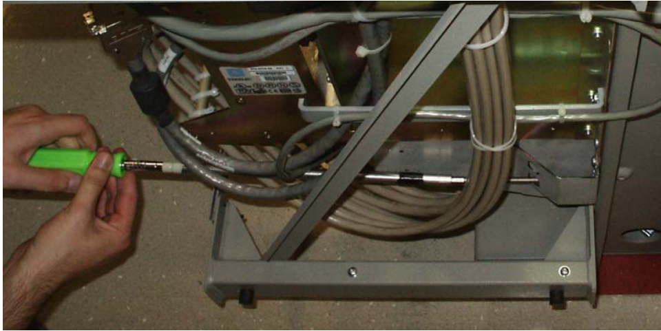
Figure 6-22 Tighten fan side bracket screws
