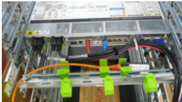
Figure 1-8 Cables Routed Through the Cable Management Arm
