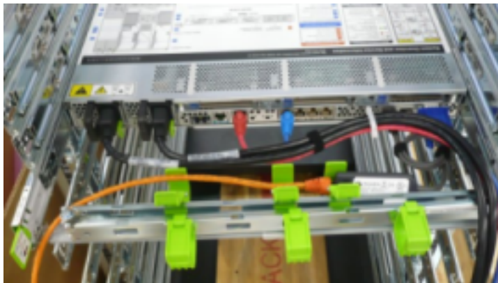
Figure 2-5 Cables Routed Through the Cable Management Arm
