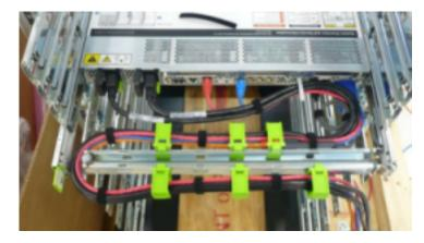
Figure 2-7 Cables Secured with Hook and Loop Straps at Regular Intervals
