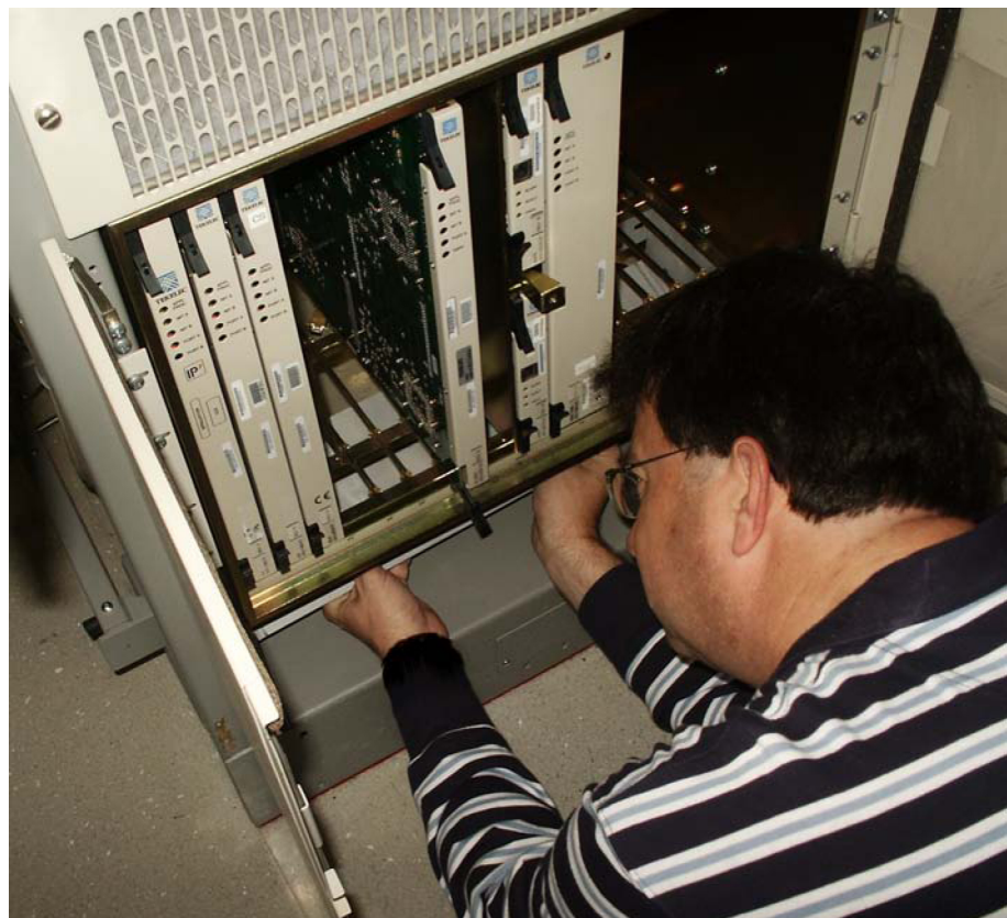
Figure 6-17 Insert fan tray bracket
