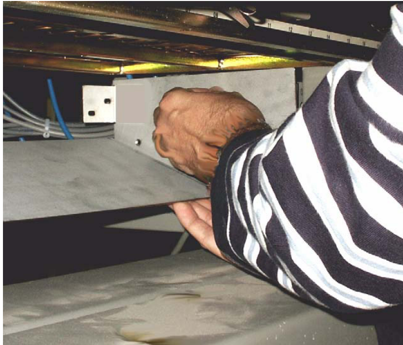
Figure 6-18 Attaching the fan tray bracket to the side brackets - inside front
