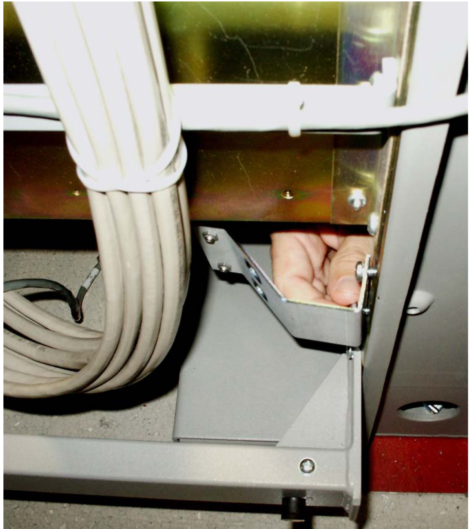
Figure 6-14 Attach side fan bracket to front frame rail
