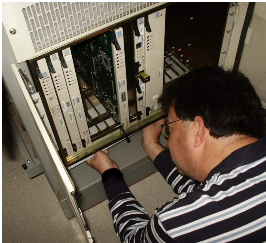
Figure 6-17 Insert fan tray bracket
