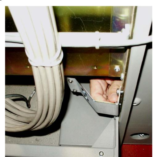
Figure 6-14 Attach side fan bracket to front frame rail
