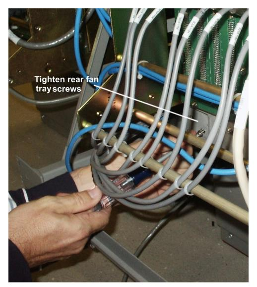
14. At this time check and tighten all screws, including the screws holding the side brackets to the frame. The side bracket screws should be tightened fully from the rear of the frame. Use a long hex driver or flat head screw driver.
